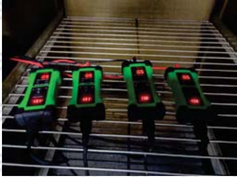
Testing-3 (Operation- function inspection)
